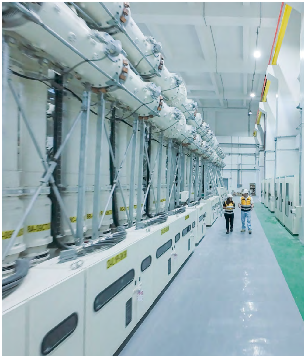
In our 585 MW SanMar Solar, we built a gas-insulated type substation with intricate engineering requirements to accommodate large amounts of renewable generation.
