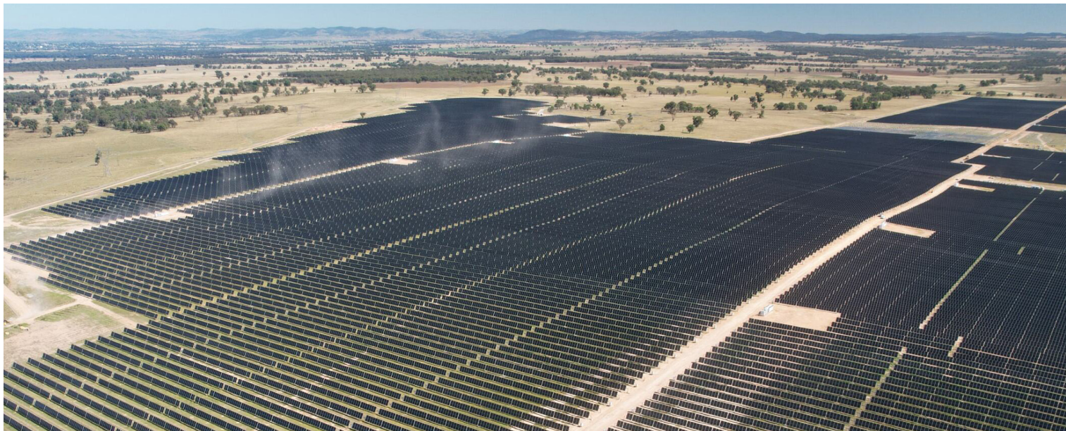
The 520 MW Stubbo Solar located in New South Wales, Australia is expected to be completed in Q3 2025.
