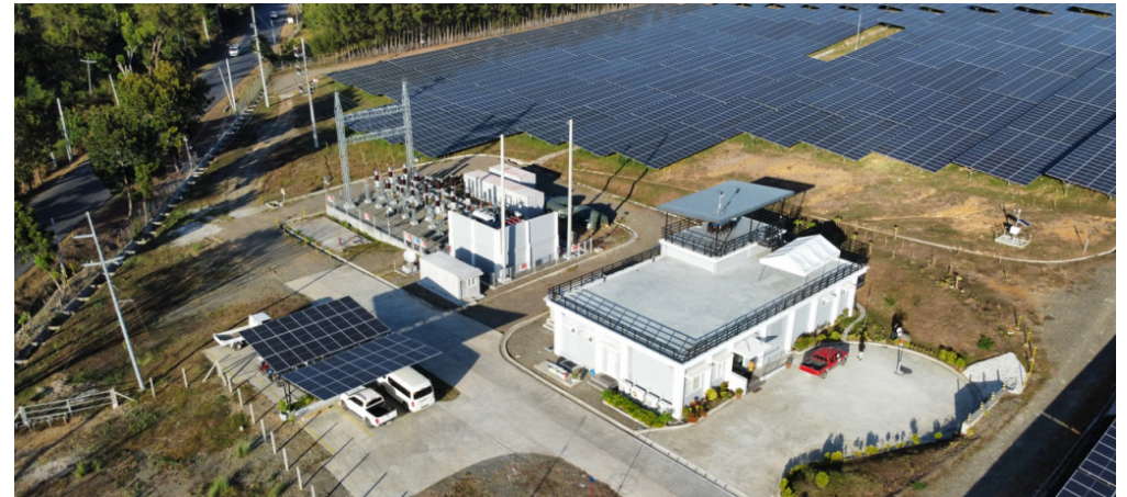
In Palauig Solar, we optimize energy efficiency by installing solar panel roofing over the control building's parking area, reducing energy consumption while maximizing clean energy use.
