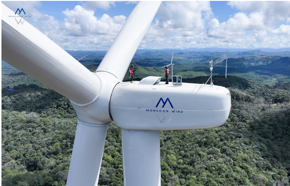
Our 600 MW Monsoon Wind project is the largest wind farm in Asia and the first cross-border wind project exporting electricity from Lao PDR to Vietnam.
