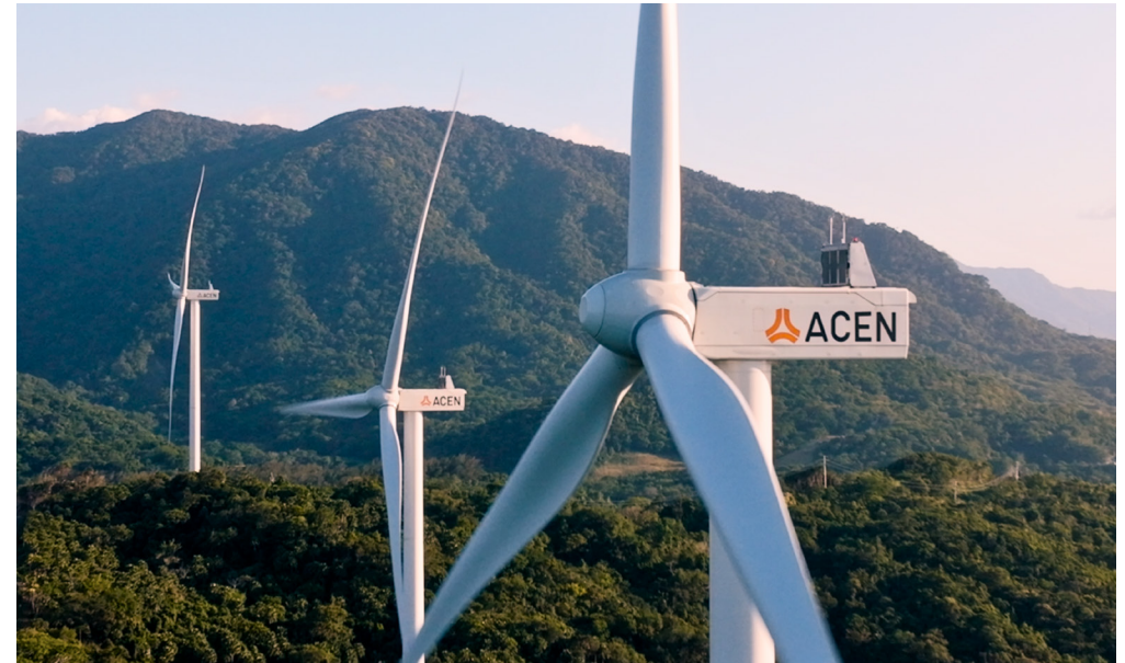
The 160 MW Pagudpud Wind in Ilocos Norte comprises 32 wind turbine generators, each capable of producing 5 MW of power.
