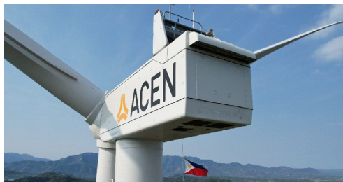
Construction for the 70 MW Capa Wind, our fourth wind project in Ilocos Norte, was completed in 2024.
