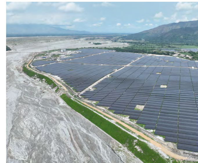
In San Marcelino, Zambales, our 585 MW SanMar Solar, which sits on over 500 hectares of idle land covered by lahar, is touted as the largest solar farm in the Philippines to date. Its third phase is expected to finish construction by 2025.
