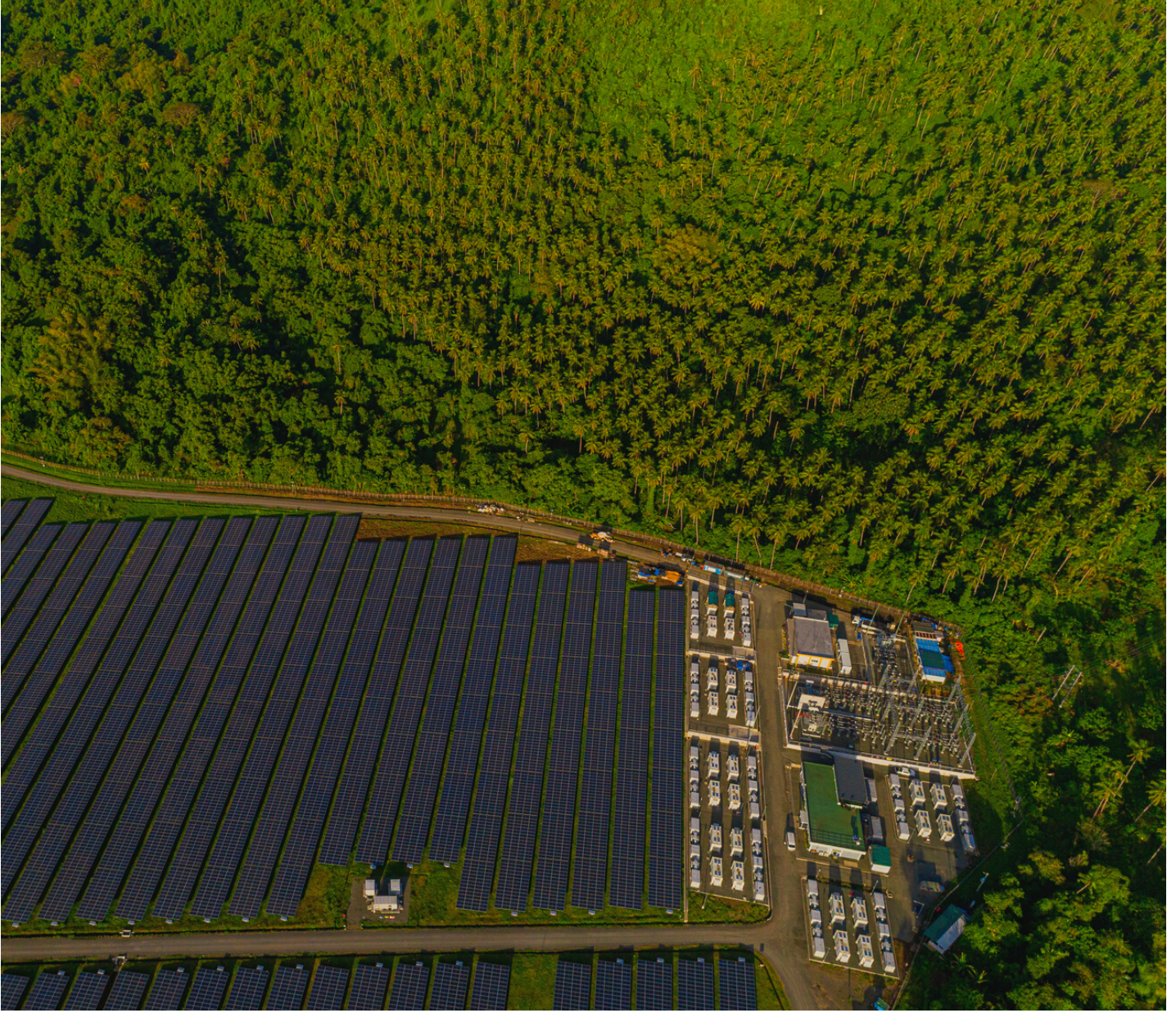
The 120 MW Alaminos Solar and 40 MW Battery Storage project in Alaminos is a hybrid development that is the first of its kind in the Philippines
