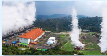
Indonesia Salak & Darajat Geothermal
